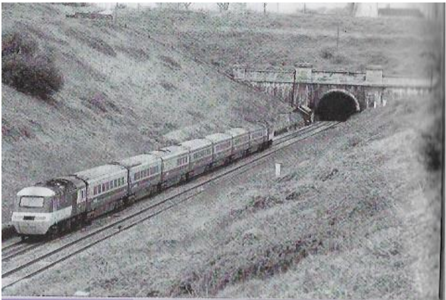
A Paddington to South Wales High Speed Train entering the Severn Tunnel
