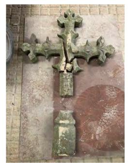
Fifteen years ago we realised that the pinnacles were severely weathered, and the east end cross was cracked. Whilst the pinnacles were wrapped in netting by Mark Hancock of Centreline (our current main contractor), the cross had to be taken down at once.
