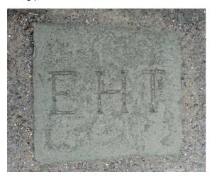
Along the route of the power cables stone tablets were installed to warn future excavators of their existence. These were engraved with the letter E.H.T., electricity high tension. Over time most have disappeared, but one still remains for us to wonder at. It may be slightly worn, but there is no reason for its removal as it maintains its purpose. Long may it stay there.
